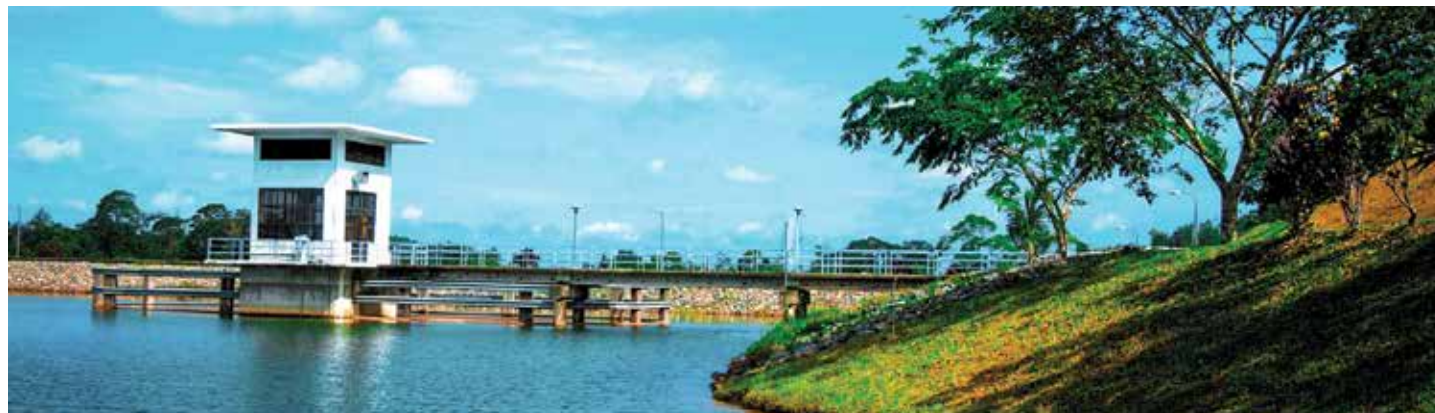
Sungai Lebam Water Treatment Plant, one of the water treatment plants that acquired OHSAS 18001.
