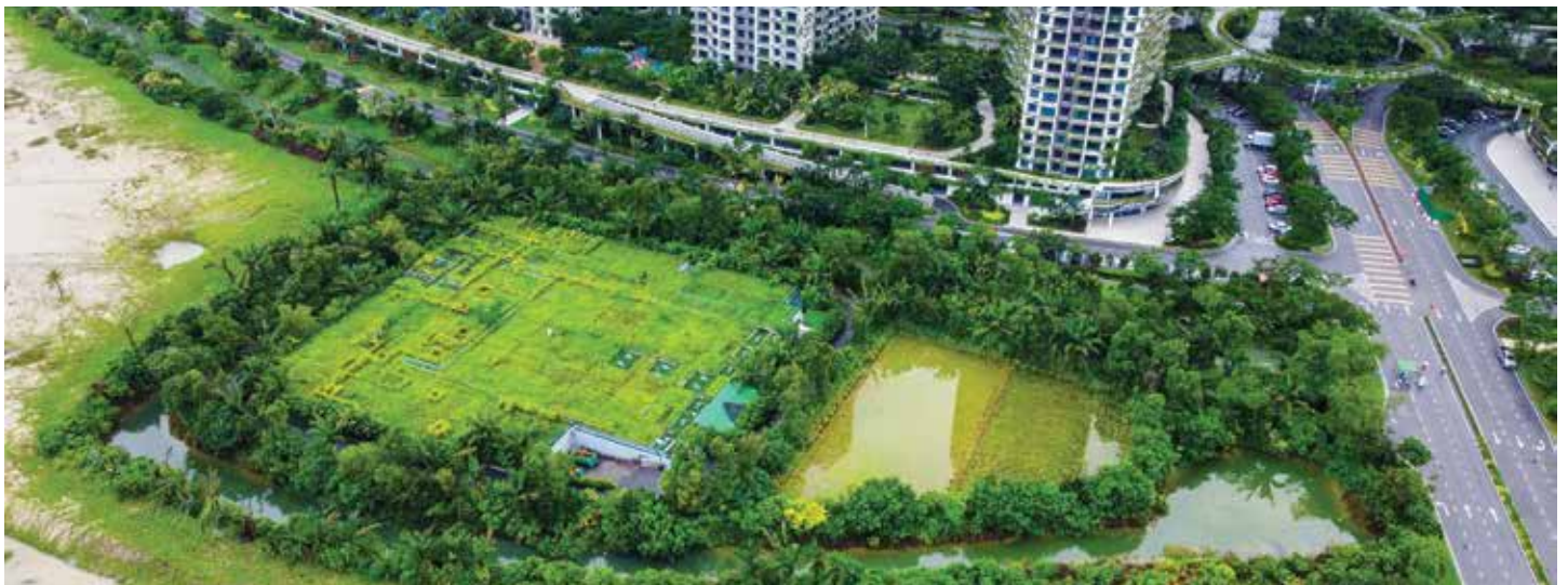
Forest City Sewerage Treatment Plant ("STP4").
