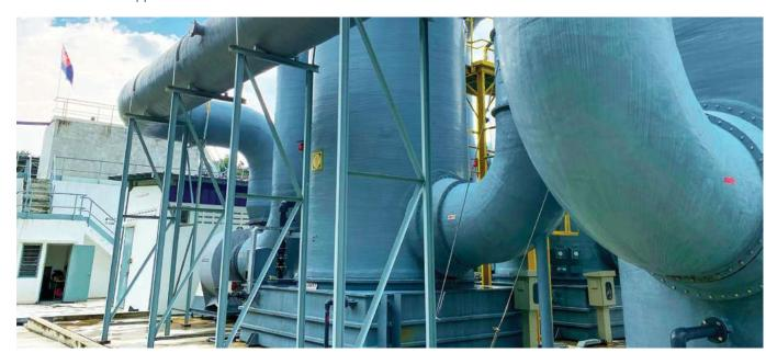
Air stripper and gas scrubber with treatment capacity up to 500 ppm of ammoniacal nitrogen content operation at Pollutant Removal System ("PRS") Simpang Renggam Water Treatment Plant
