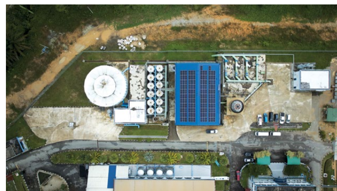
Ranhill's 54 kWp Solar PV System at the 20 MLD Sultan Iskandar WTP Extension Project
