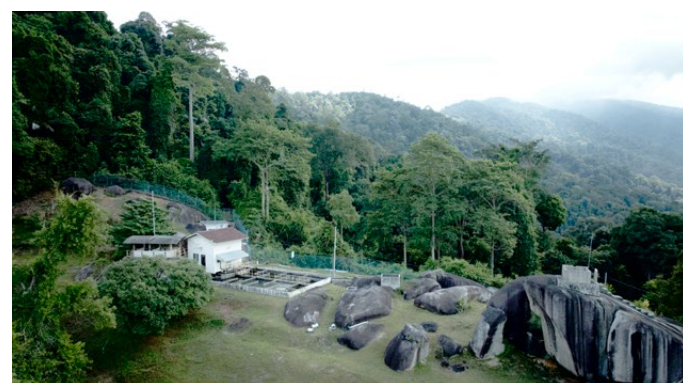
Micro Hydro Application at Gunung Ledang Water Treatment Plant, Tangkak, Johor
