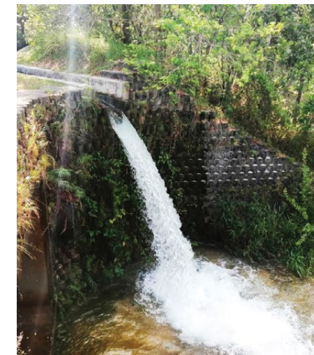
Outfall at Layang Dam from Tasik Biru raw water pumping system
