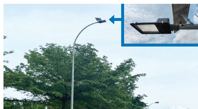
Replacing traditional street lights with solar-powered street lights at most WTPs
