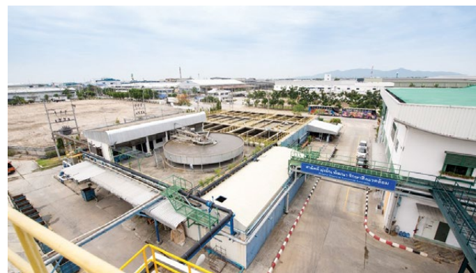
RWT's Wastewater Treatment Plant in Chonburi, Thailand
